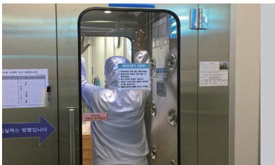
Air Shower Room
